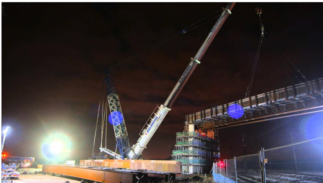
Figure 26 Bridge Lift over ECML, Doncaster
