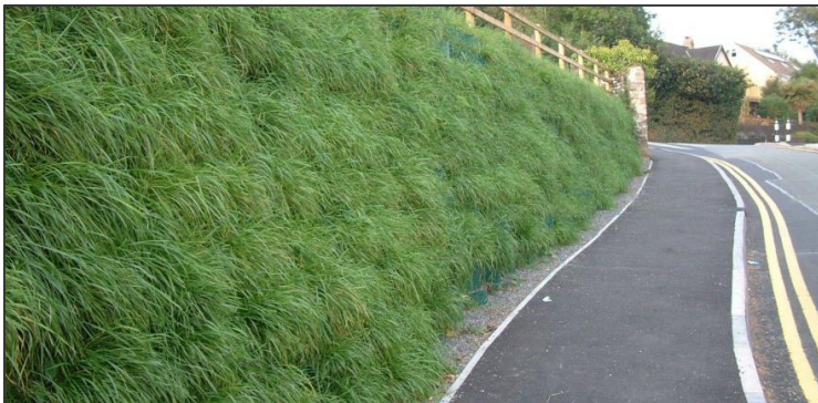
Figure 16 Example of Reinforced Earth Retaining Wall with Vegetated Face
